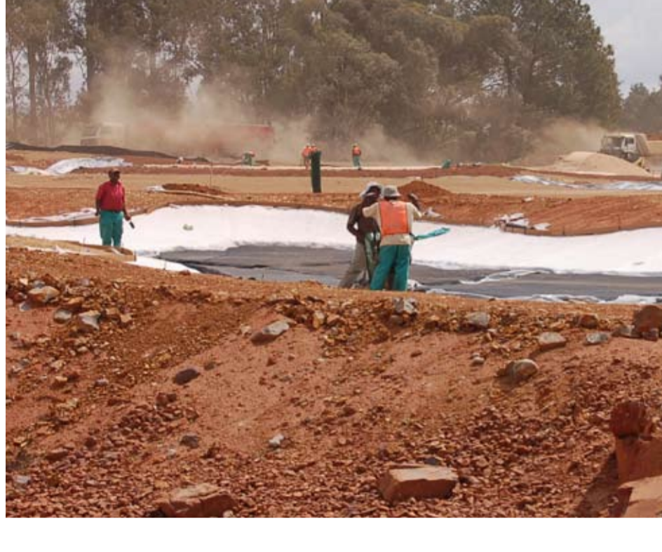
ABOVE Lining of bunker on 2nd hole
